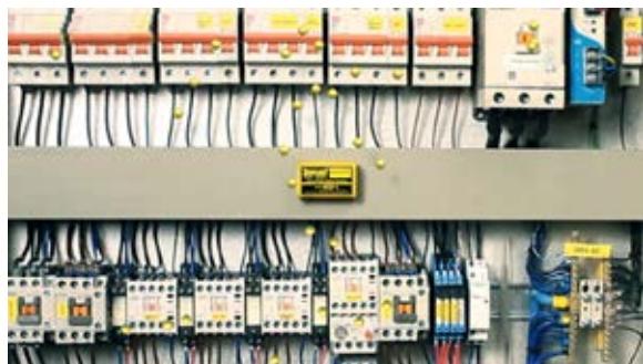
Zerust corrosion inhibitor diffusers go to work in minutes to saturate enclosures with protective VCI molecules.
