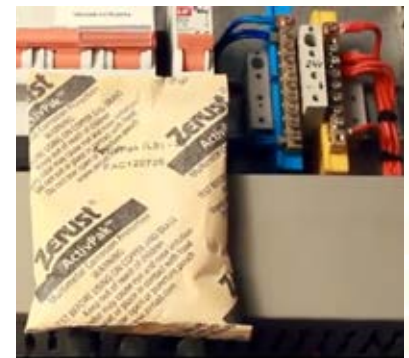
ActivPak(LS) diffuser packet protects in corrosive environments.
